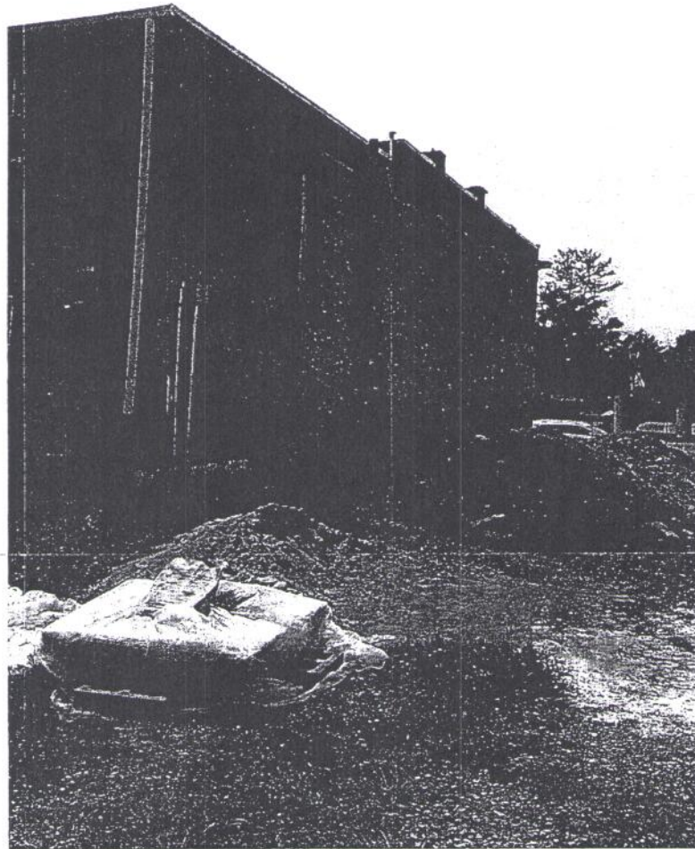
Exterior West brick wall
