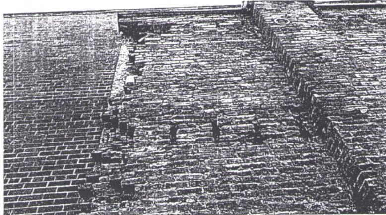
Pockets for joist seats, of the removed building
